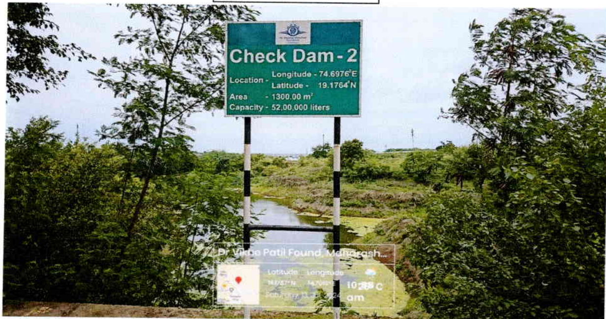
Check Dam No -2
